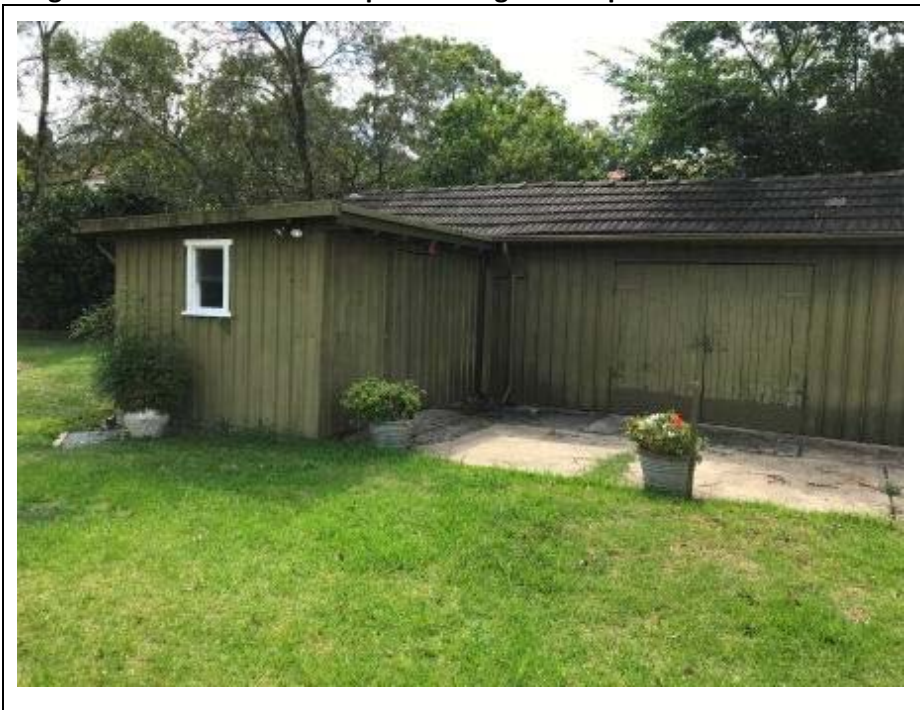
Image 6.2.7 View of northern portion of greenkeeper sheds
