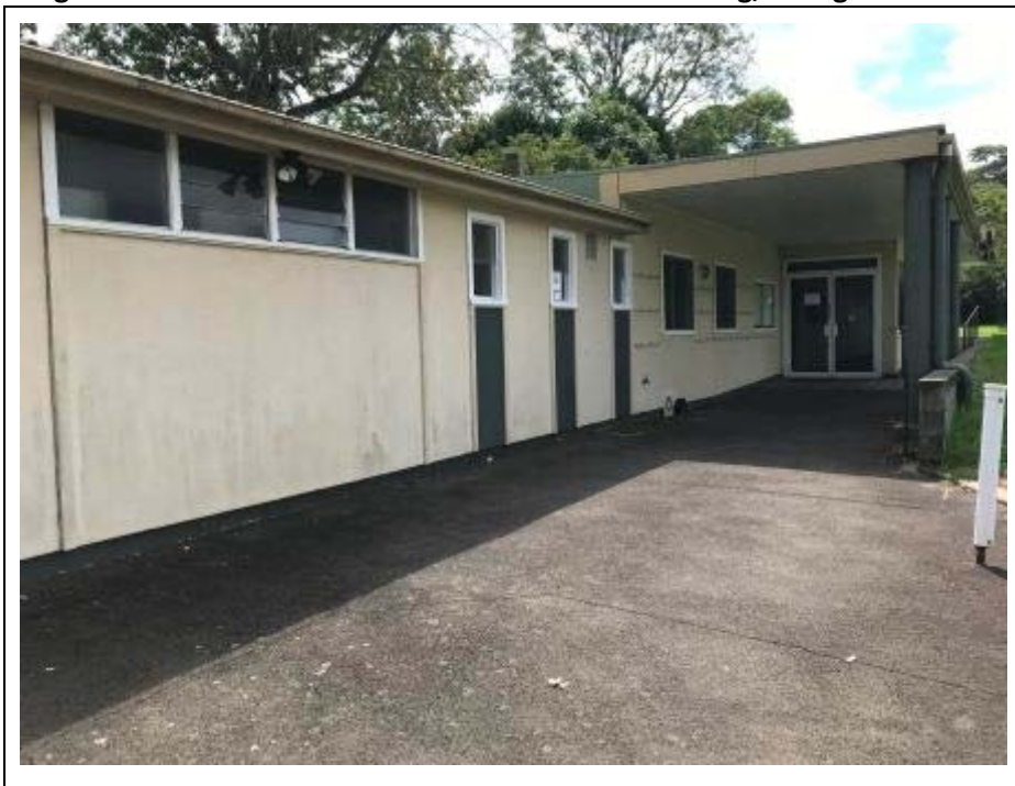
Image 6.2.1 View of southern side of clubhouse building, facing north east
