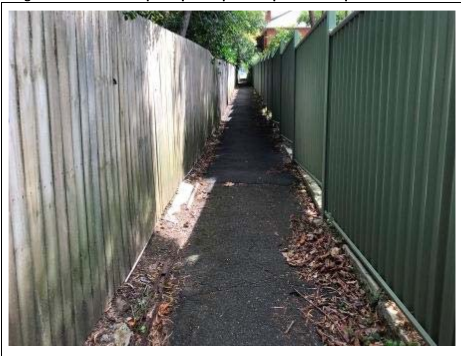
Image 6.2.11 View of asphalt paved path on pan handle portion of site
